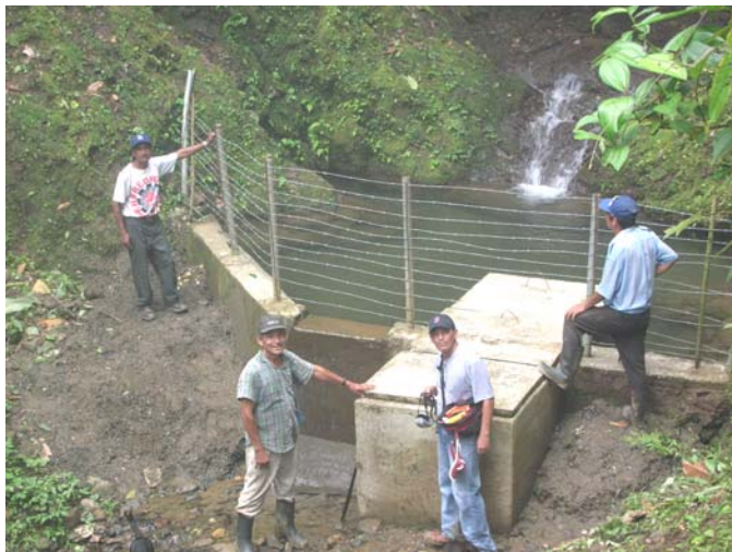
Source for Nueva Vida water system
