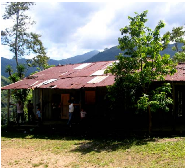
Chachaguala Arriba school (before rehab)
