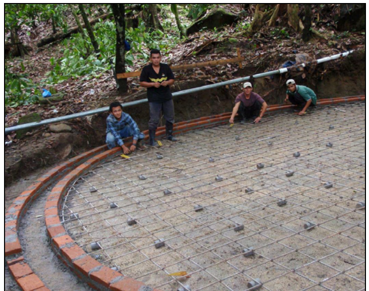
BASE OF NEW TANK UNDER CONSTRUCTION
