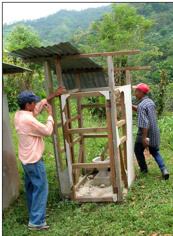
BEGINNING THE REBUILDING OF EARTHQUAKE-DAMAGED LATRINES
