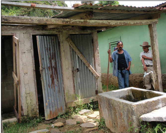
RECONSTRUCTION OF LATRINES IN NUEVA PALMAS REAL
