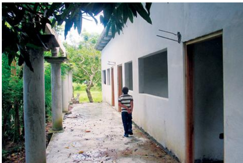
Claudio, a Milla Cinco student, inspecting his (almost) new home...
