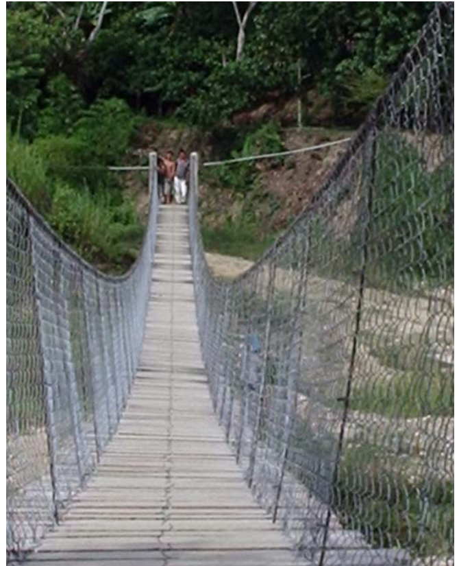
New bridge over Rio Omoa
