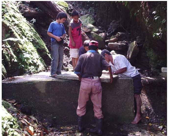
The small dam that impounds water to supply the Las Flores system
