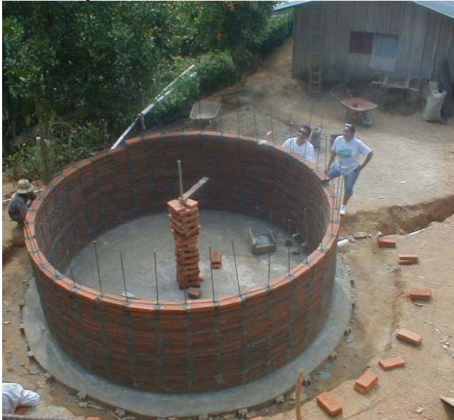
Water tank under construction in Las Brisas de Rio Negro
