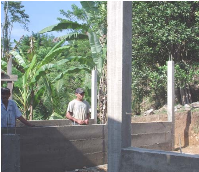
Chachaguala Arriba school construction in progress.
