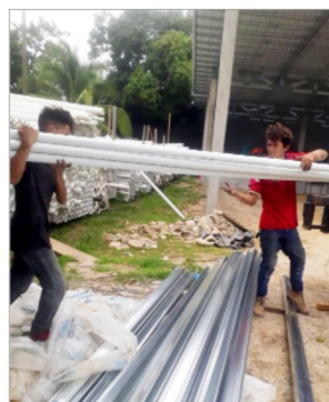
Tubes being delivered for the Nueva Esperanza water system.
